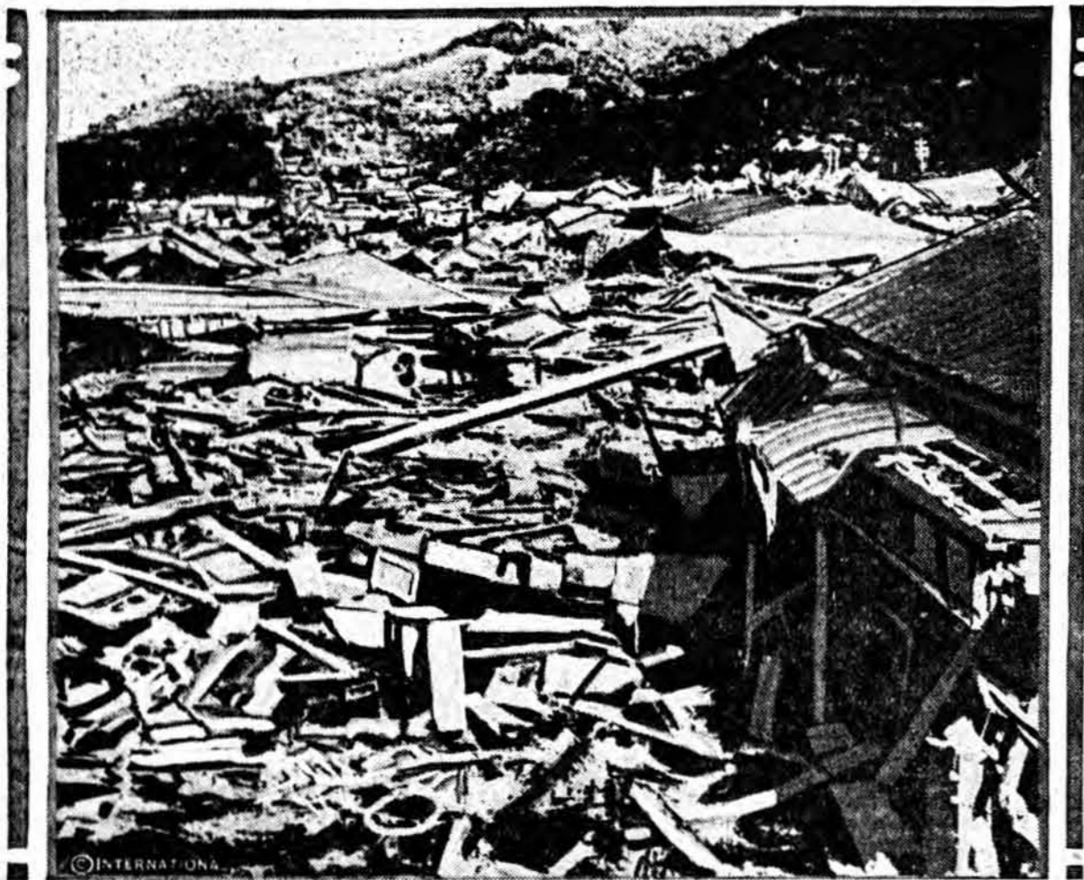
This expanse of tangled wreckage was all that was left of Ito, a busy town in Idzu prefecture, after the earthquake and fire had done their work.
