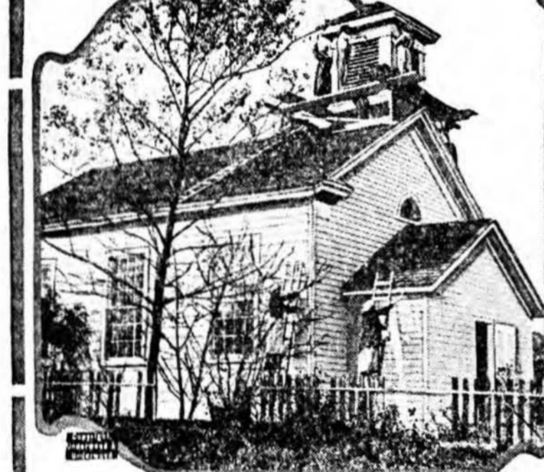
When recently it became necessary to have the Unionsdale chapel at East Hempstead, Long Island, repainted the painters wanted too much for the job. So members of the ladies' aid society decided to do the work themselves. Seventeen of them put on overalls and speedily painted the chapel.
