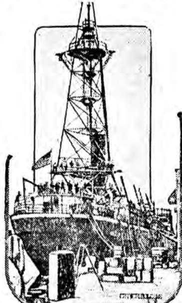
The dirigible mooring mast being moved aboard the U. S. S. Patoka at the Norfolk navy yard, Norfolk, Va. The Patoka is the first ship in the United States navy to be equipped to handle dirigibles.
