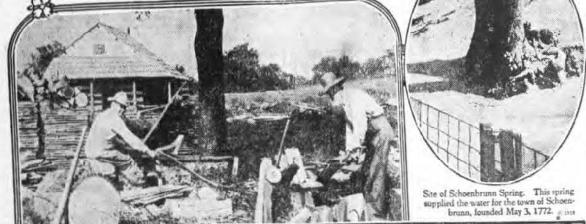
Splitting and shaving shingles—pioneer style—for school house, Sept.-Oct., 1927. Schoenbrunn Memorial Park, near New Philadelphia, Ohio.
